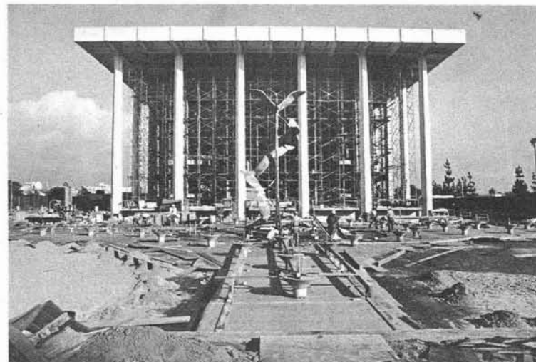
NEW AUDITORIUM PROGRESSES — Construction on the new Auditorium going up on the Pasadena campus is continuing to progress toward an early-April, 1974, opening date. The men shown in the picture are working on the pool which is to surround the Auditorium. [Photo by Ken Evans]
